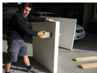
Foam is easily cut with a panel saw
