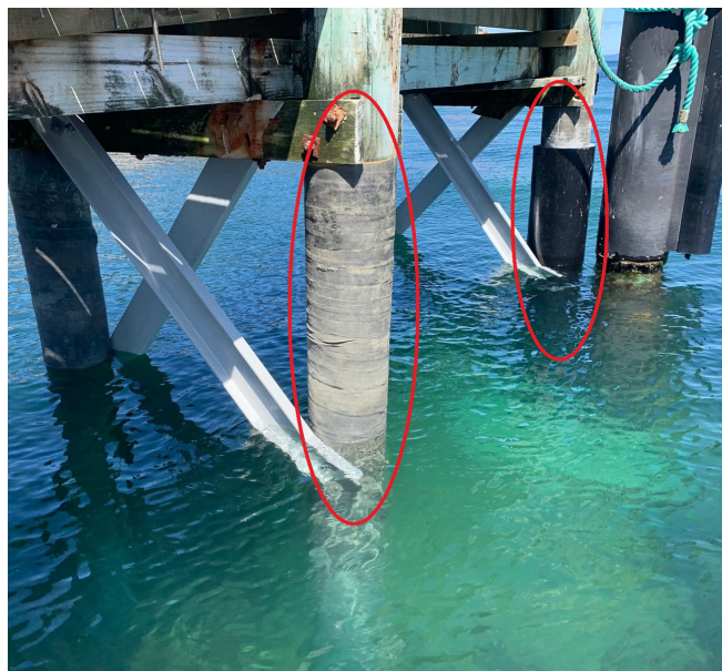
Typical timber pile repairs – fibreglass wrap in the foreground and HDPE pile jacket with grout annulus in the background
