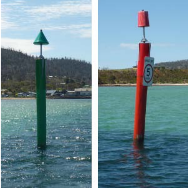
New Starboard and Port Piles Norfolk Bay
