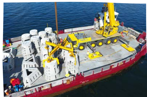
Installation of concrete reef modules
