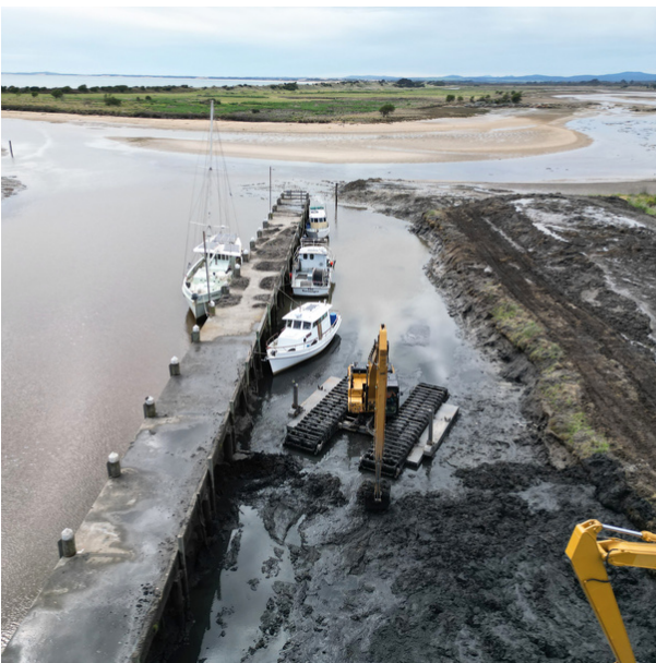
Sediment removal from behind jetty, with main berthing face already completed
