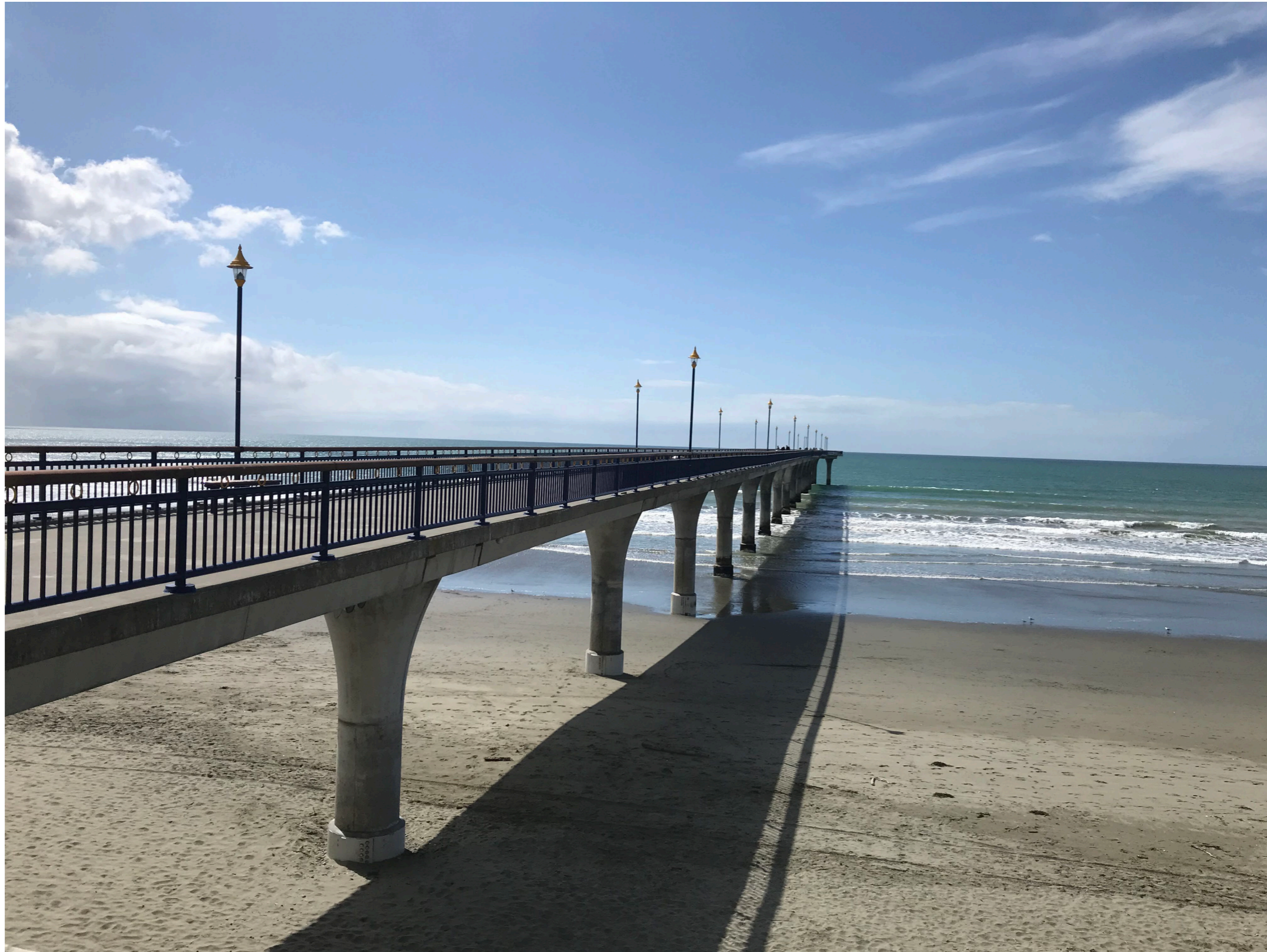
A PIER ON MAINLAND AUSTRALIA SHOWING EXAMPLES OF LIGHTING AND HANDRAIL
