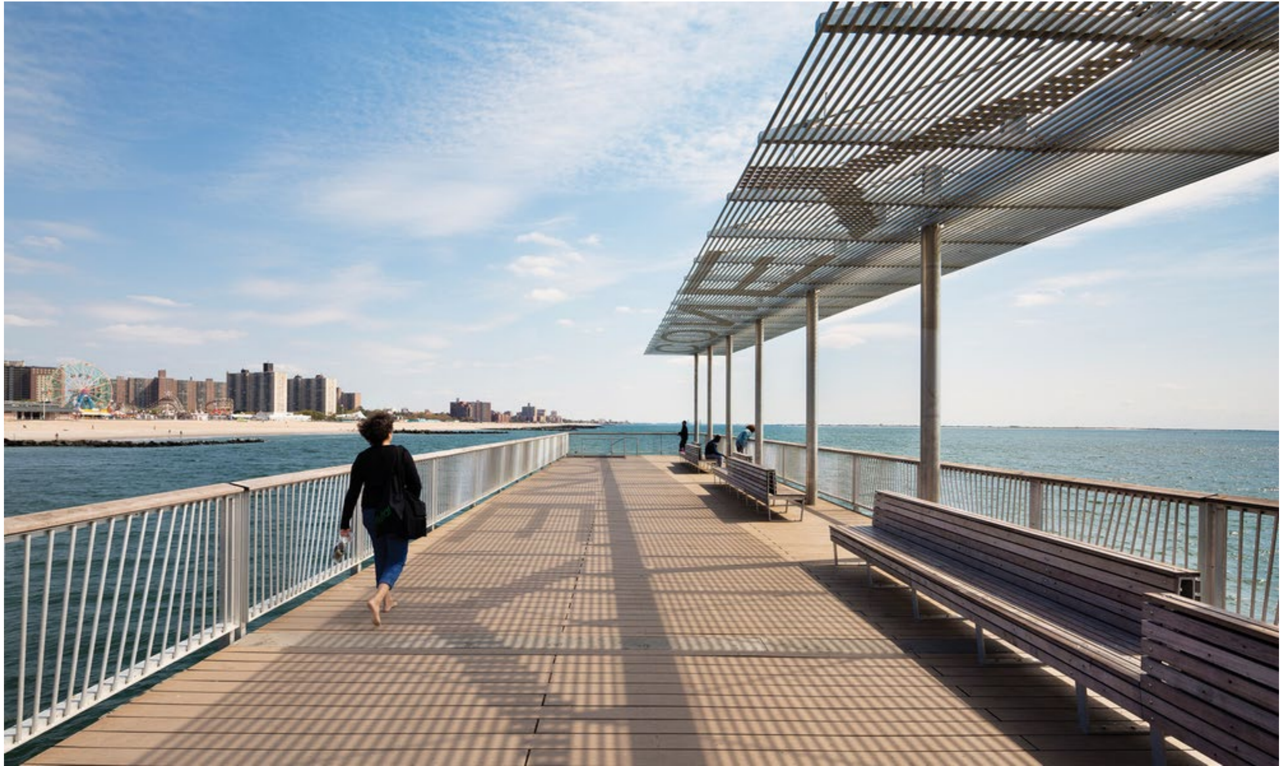
A PIER SHOWING EXAMPLES OF SEATING AND COVER
