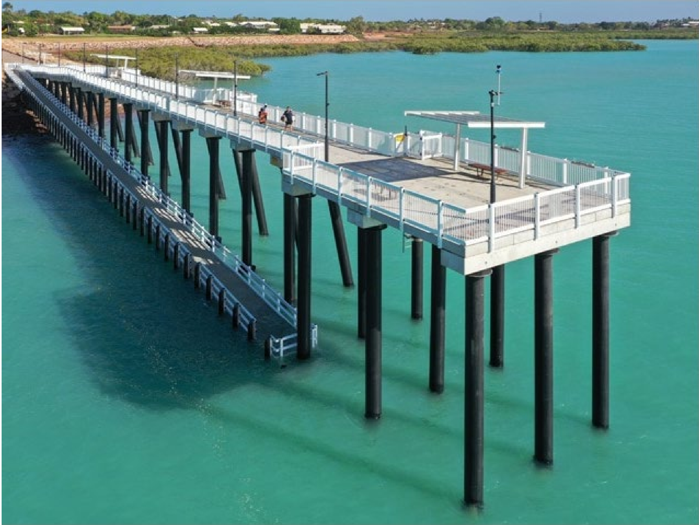
EXAMPLE OF A PIER FROM WESTERN AUSTRALIA HIGHLIGHTING AN OPTION FOR WATER ACCESS
