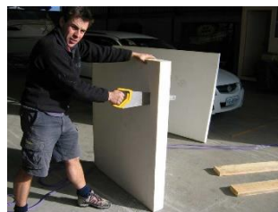
Foam is easily cut with a panel saw
